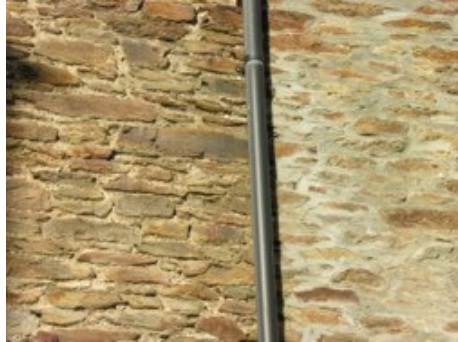
25: Bad cement pointing is ugly and harmful
